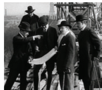
Frame from "Slotsarkitekt Thorvald Jørgensen paa Kristiansborg Slots Stilladser" / Architect Thorvald Jørgensen on the Scaffolding of Kristiansborg Castle, 1913. Politiken.
